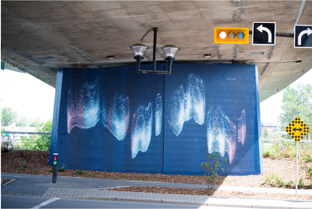
Abutment B (middle), facing south
