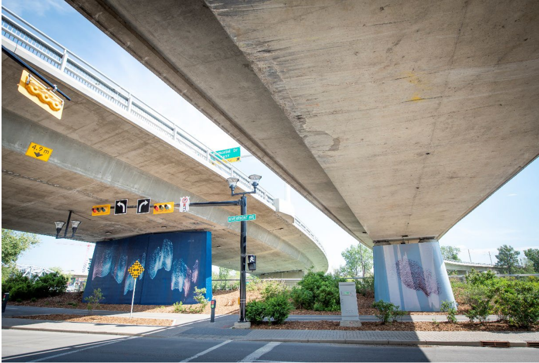
Abutment B + C, facing south
