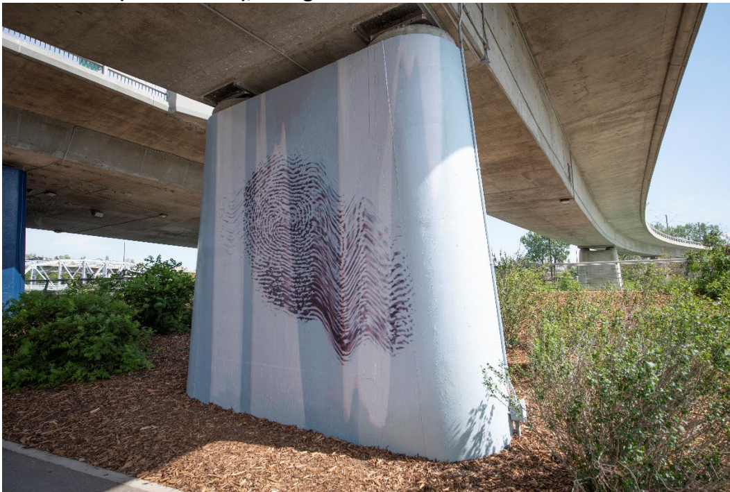
Abutment C (easternmost), facing south
